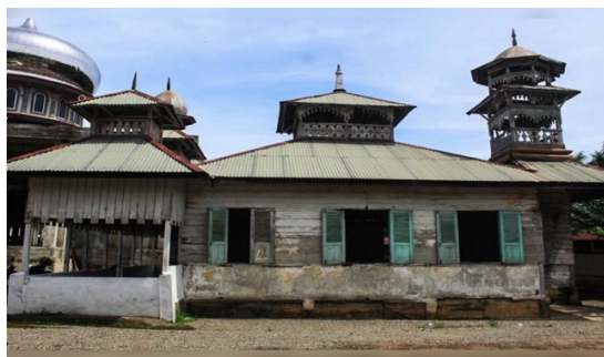
Gambar 9. Tampak Samping Masjid Tuha Gunong Kleng
